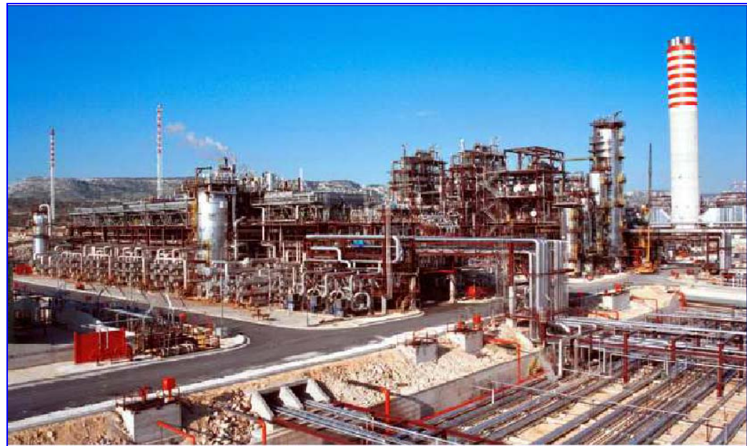
ISAB IGCC Plant
